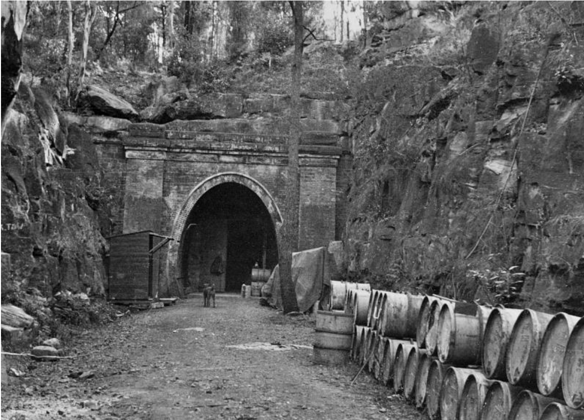
Glenbrook Tunnel, circa 1944. Photo supplied by Geoff Plunkett.
